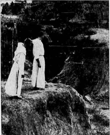
FAMOUS STREET—Two unidentified Franciscans, above, gaze at one of Santarem's famous streets. Little or practically nothing is done to maintain the streets. Above the erosion is evident. Whole houses have collapsed into the street. It is not unusual for streets in Santarem to change their course over night during the rainy season.
